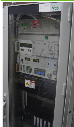
A modern solid state (transistor) pre-driver and a new Low Level RF control unit (LLRF) were installed together in the PLC cabinet (left picture).
